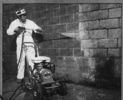
An Adjustable Pressure Washer — capable of pumping muddy water and detergents.
